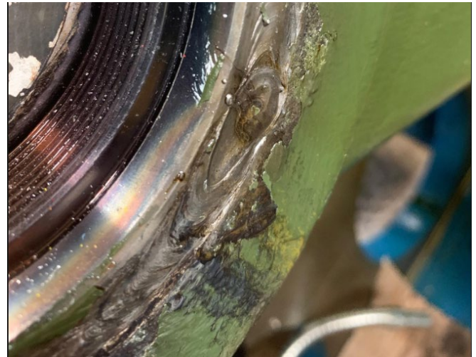
Figure 9: Baseline Weld Cracking
